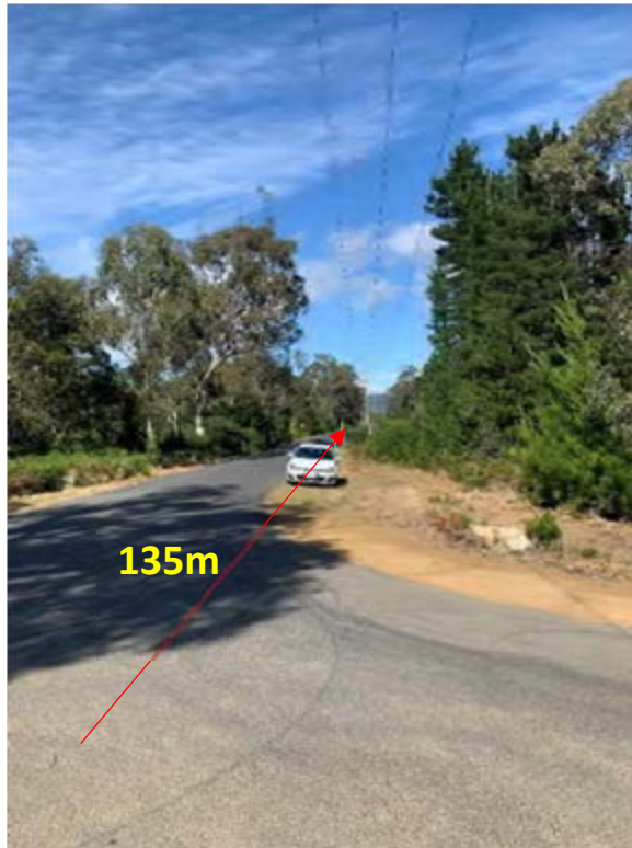
Figure 31: Sight Distance at Surf Road/Pittwater Road intersection was measured to be 135 metres to the right (West).
