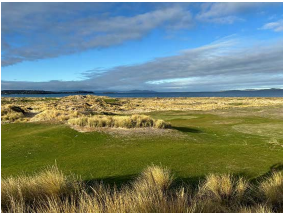
Photo 2: The Seven Mile Golf Course currently under construction
