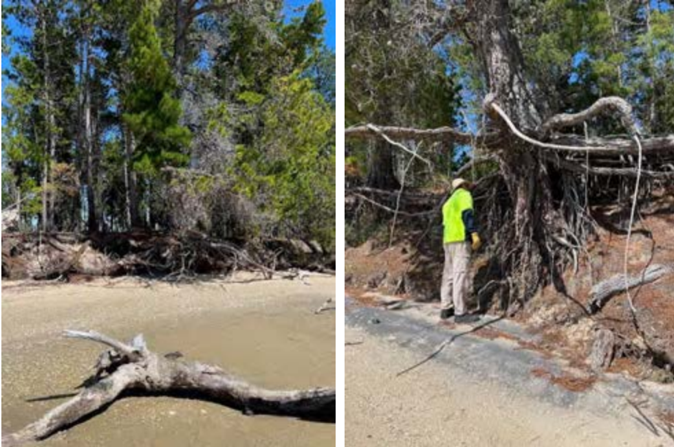
Figure 4. Site photos showing erosion along shoreline.
