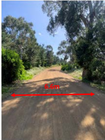
Figure 6: Photograph showing Surf Road 6.6-metre cross section width.
