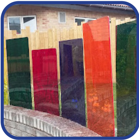
Feature Fence Steel post & wire fence with colourful plexiglass sheets for transparent wind protection. Posts can be powdercoated for pops of colour. Posts behind goal posts could have chainwire mesh for ball rebound net
